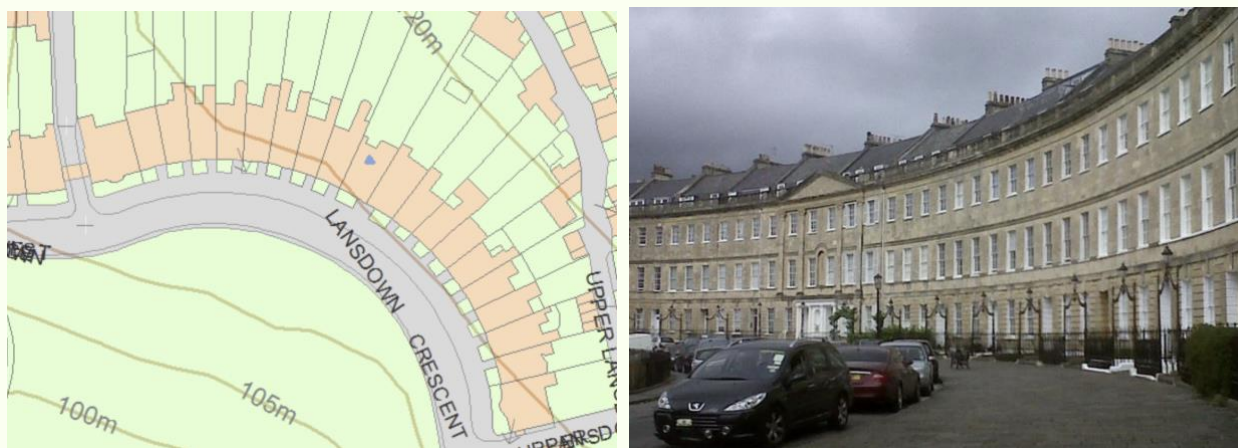
Figure 1: The list entry for Grade I 1-20 Lansdown Crescent in Bath covers 20 terraced houses. Source: Historic England ( https://historicengland.org.uk/listing/the-list/list-entry/139410 ).
