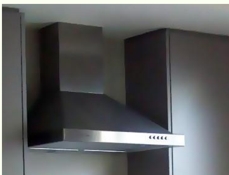
Kitchen hood extractor fan
