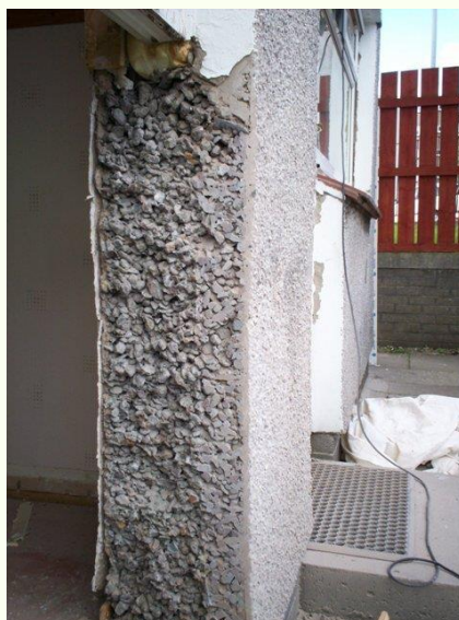
Figure 1: A cross section of a no-fines wall. Source: Non Standard House Construction
