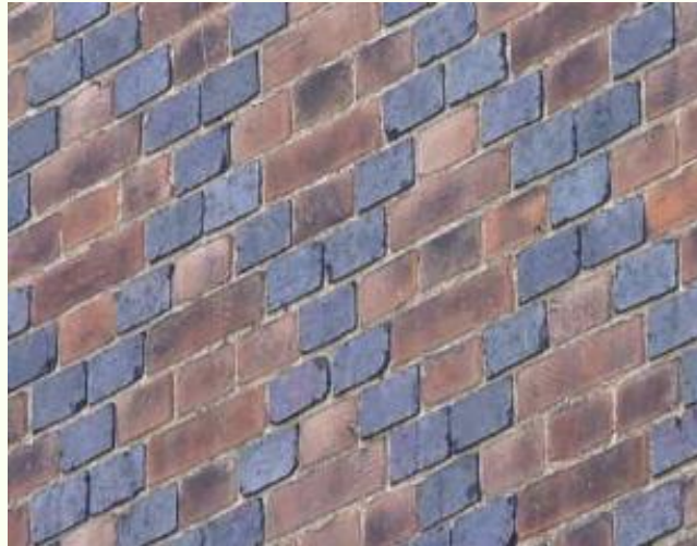
Figure 1 shows a solid brick wall. Most of the bricks are laid as 'stretchers', so their long side can be seen from the front, but the blue 'header' bricks are perpendicular to that and tie the two leaves of adjacent brickwork together.
