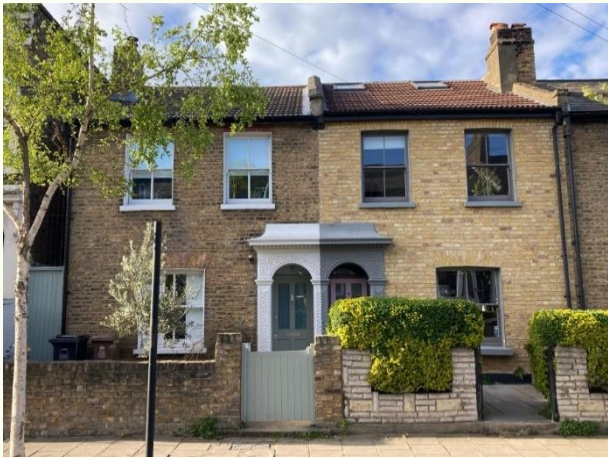
Figure 1: Two London yellow stock brick homes in London, with one recently sandblasted. Source: Building London
