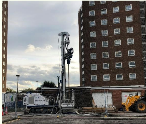
Figure 5 shows ground source heat pump installation in Thurrock. Source: Baily Garner LLP
