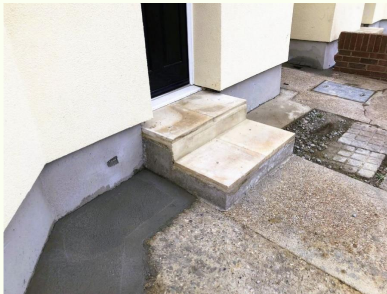
Figure 1 shows a thermally broken step as part of external wall insulation in Havering, which is a detail that PAS 2035 processes seek to guarantee. Source: Baily Garner LLP
