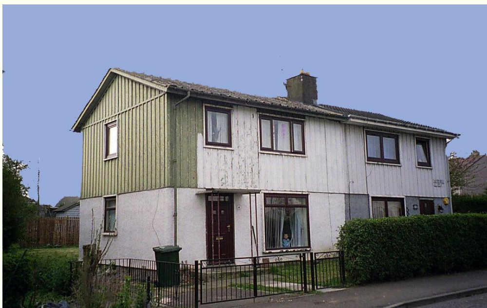
Figure 2 shows a BISF property with its original asbestos roof and awning over the door. Source: strutherm.co.uk
