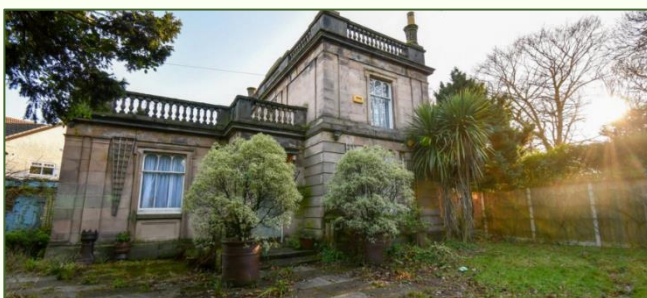
Figure 6 shows Central Lodge, a vacant building in Birkenhead registered park, which is being currently being retrofitted. Source: Ecospheric
