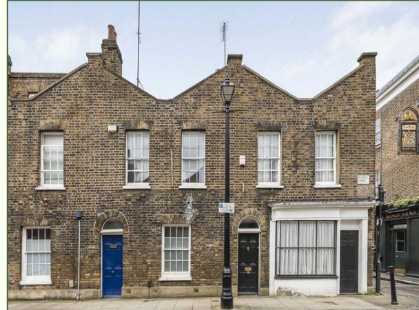
Figure 3 shows 1 – 9 Theed Street, London, a row of nine homes covered by one listing. Source: Prime Location
