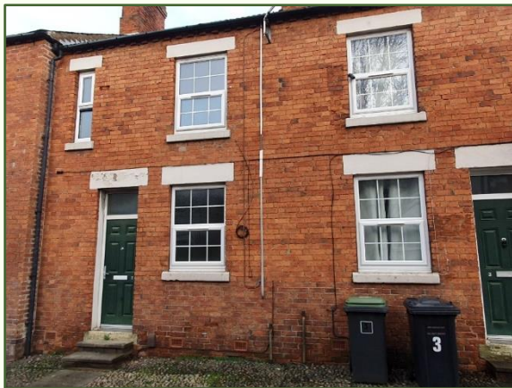
Figure 4 shows social housing in Eastwood conservation area, Broxtowe. Source: Broxtowe Council
