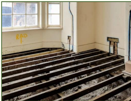
Figure 3 shows a suspended timber floor without floorboards. These were developed to avoid damp problems associated with laying floorboards directly on solid ground. Source: Ecological Building Systems
