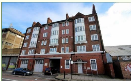
Figure 4 shows a former fire station in Tower Hamlets, which was converted into housing in 1997. All the windows and doors would have originally been timber with single glazing. Source: Historic England.
