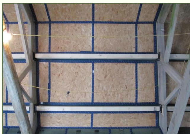
Figure 16 shows airtightness tape between insulation boards in the roof of a historic building. Source: 21degrees.com
