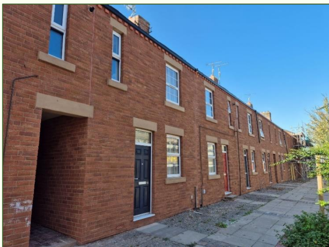
Figure 13 shows art brick EWI used in a conservation area. Source: Broxtowe Council
