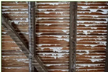
Figure 6 shows the reverse of a lathe and plaster wall, which from the front appears smooth. Source: Historic England
