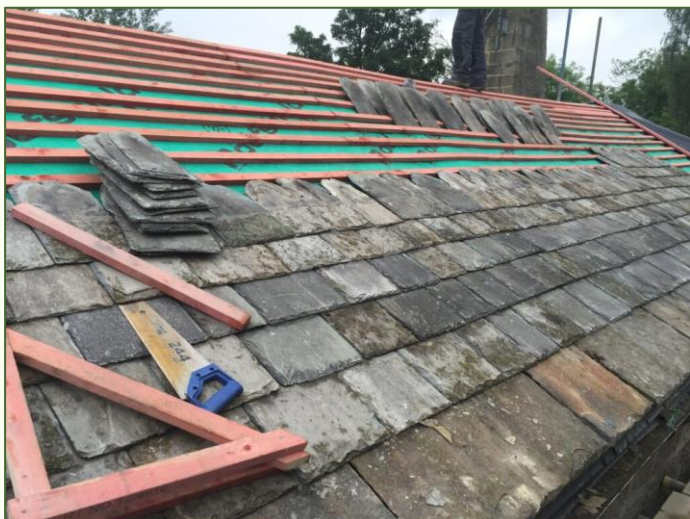
Figure 8 shows a pre-1919 building being reroofed with Westmorland slates. Source: nealroofing.com
